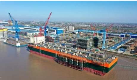
FPSO : Moving to site
